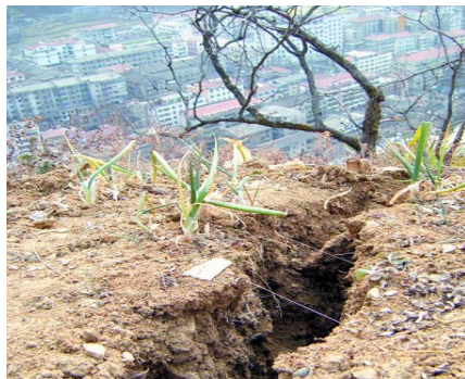
Figure2: Ground fissure because of landslides
